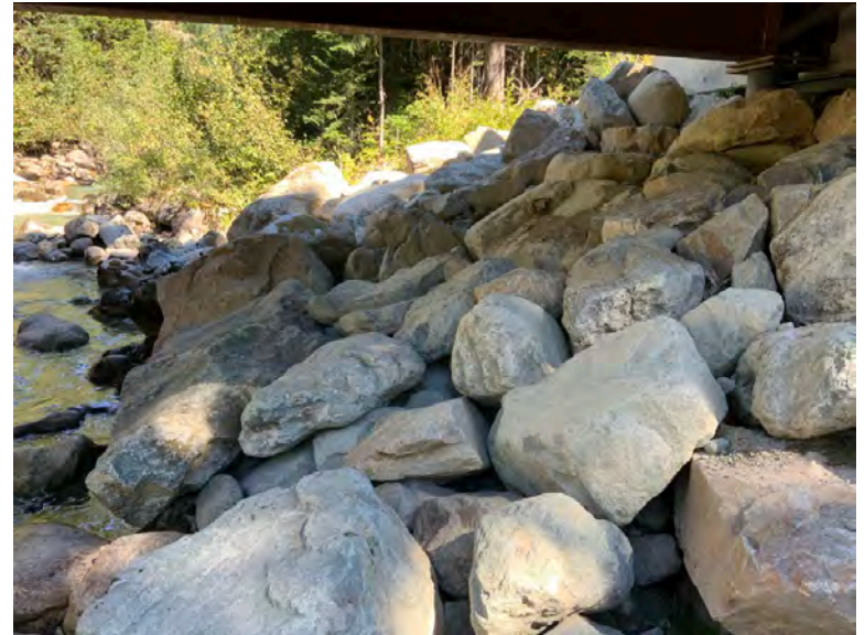
Left Bank Abutment when facing downstream
