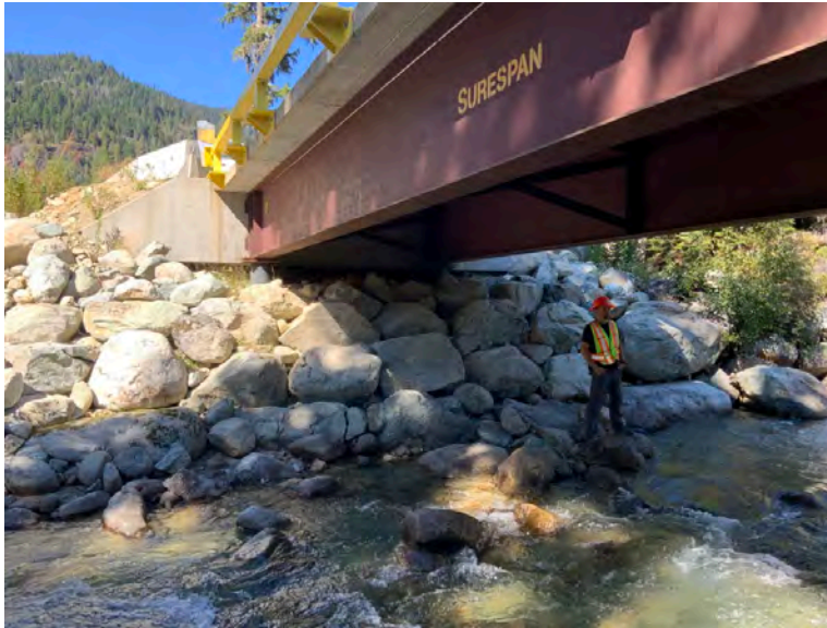
Right Bank Abutment when facing downstream
