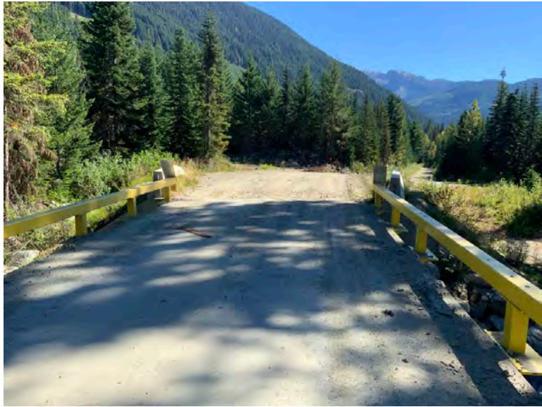
Approach from Left Bank when facing downstream
